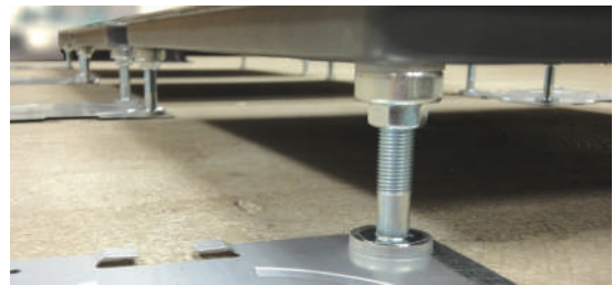
step 1 and 3: loose and fasten the pedestal at the lock-nut at bottom
